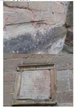
Priest's Vestry – The east gable stonework and pointing in fair condition with some individual stones weathered, some open jointing and moss/vegetation at plinth level. As elsewhere, cement pointing is aggravating damp and deterioration. The stone tracery of the window appears sound.
